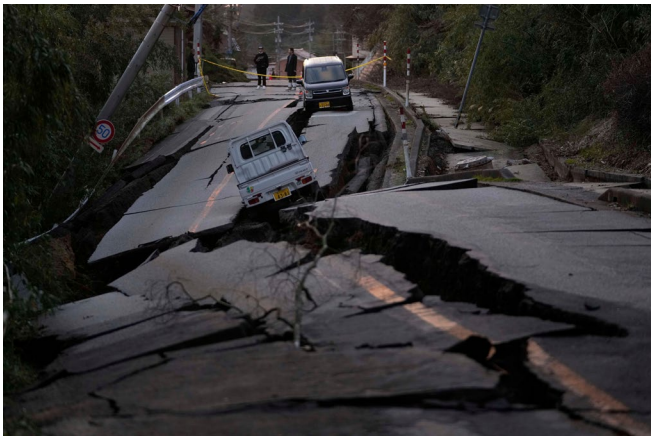
Figure 1. Aftermath of the 2024 Noto earthquake, northwest of Tokyo. The powerful quake severely cracked roads and caused heavy damage to infrastructure, leading to massive disruption in emergency response.
